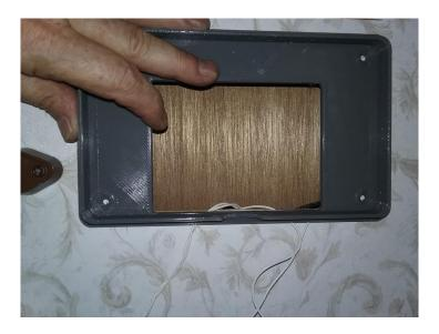
1) TEST FIT - Verify the opening in the wall is at least the same size as the opening in the back of the wall plate.
