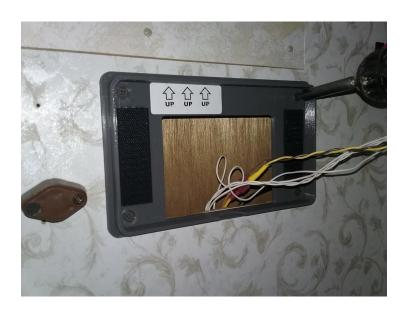
2) SECURE PLATE TO WALL - Ensure the wall plate is oriented with the TOP side up. Level the wall plate over the opening and install the four #8 screws. If the screws are going into a thin wall, you can use the metal speed nuts on the inside of the wall, but make sure the wiring doesn't get pinched between the speed nuts and the wall..
